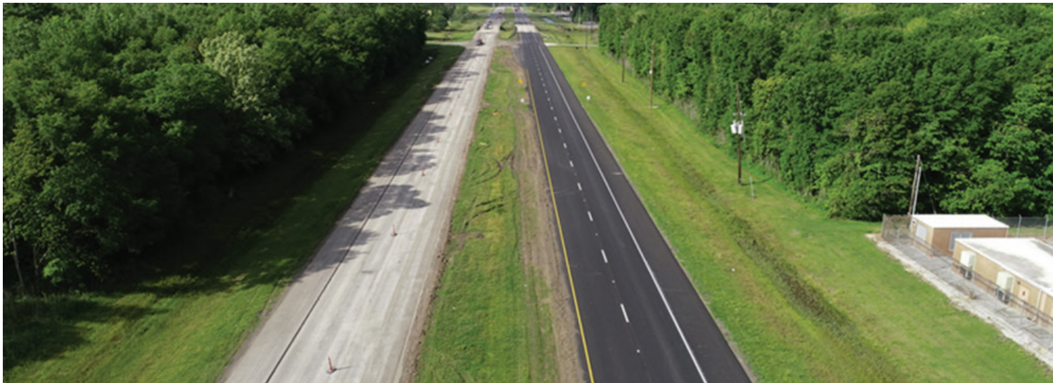
PHOTO DURING CONSTRUCTION OF LA 22 REHABILITATION PROJECT
